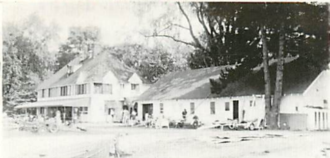
CLYC Clubhouse showing sail and locker rooms on the right.
