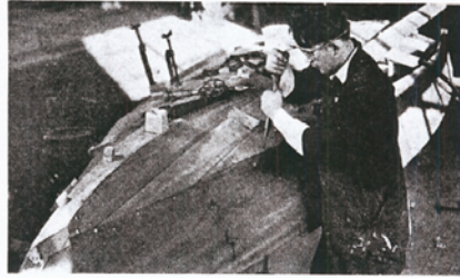
25—Bottom planks screwed to frames
