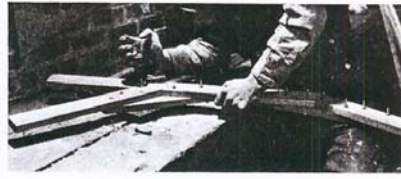
5—Cutting off excess copper rivet
