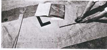
1—Laying down lines of Snipe from table of offsets
