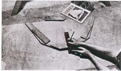
2—Checking frame one and marking in center line
