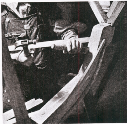
17—Second operation of number 16. Chine pieces are also set in stem
