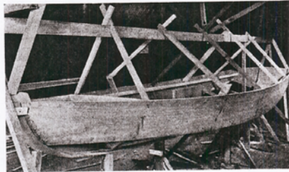
21—Side planks complete
