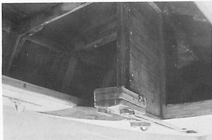
Before: View of original construction with dagger board trunk at deck level.
