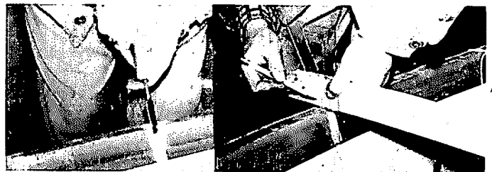
Notching the clamp.
