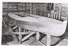
Top: One of the many Snipes being built at Trenton, Ontario
