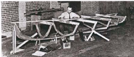
Below: Snipe No. 6 being built by E. B. Montgomery of the Dallas Sailing Club. Right: No. 8, owned by F. L. Weckman of Jamestown, New York
